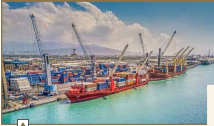
KWL's Terminal now operates 24 hours per day, 365 days per year with a quay 1,655 metres long, offering 9 deepwater berths with draft up to 13 metres for ro-ro, lo-lo, container, general break bulk and bulk cargoes.
