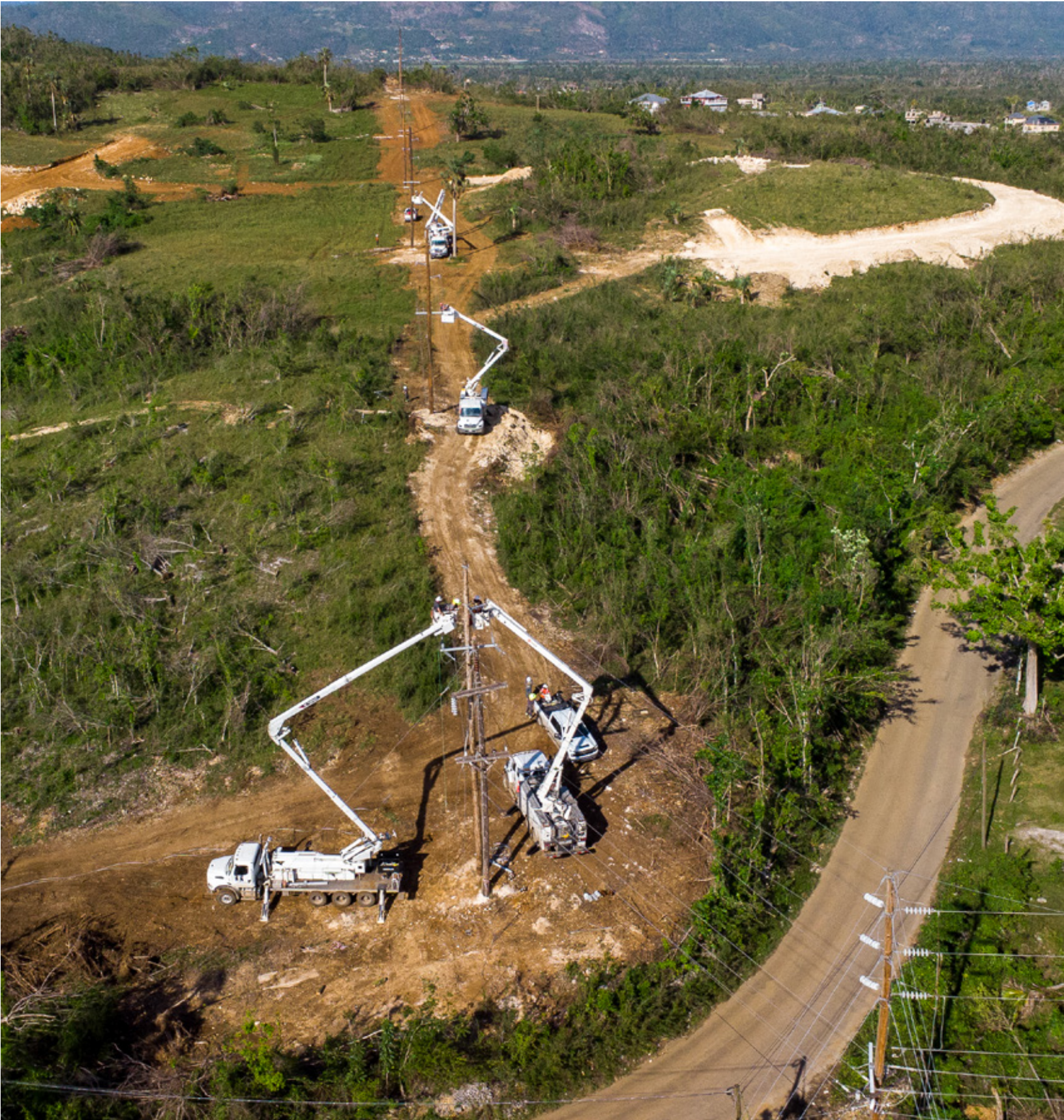
Restoration work in progress in Santa Cruz, St Elizabeth
