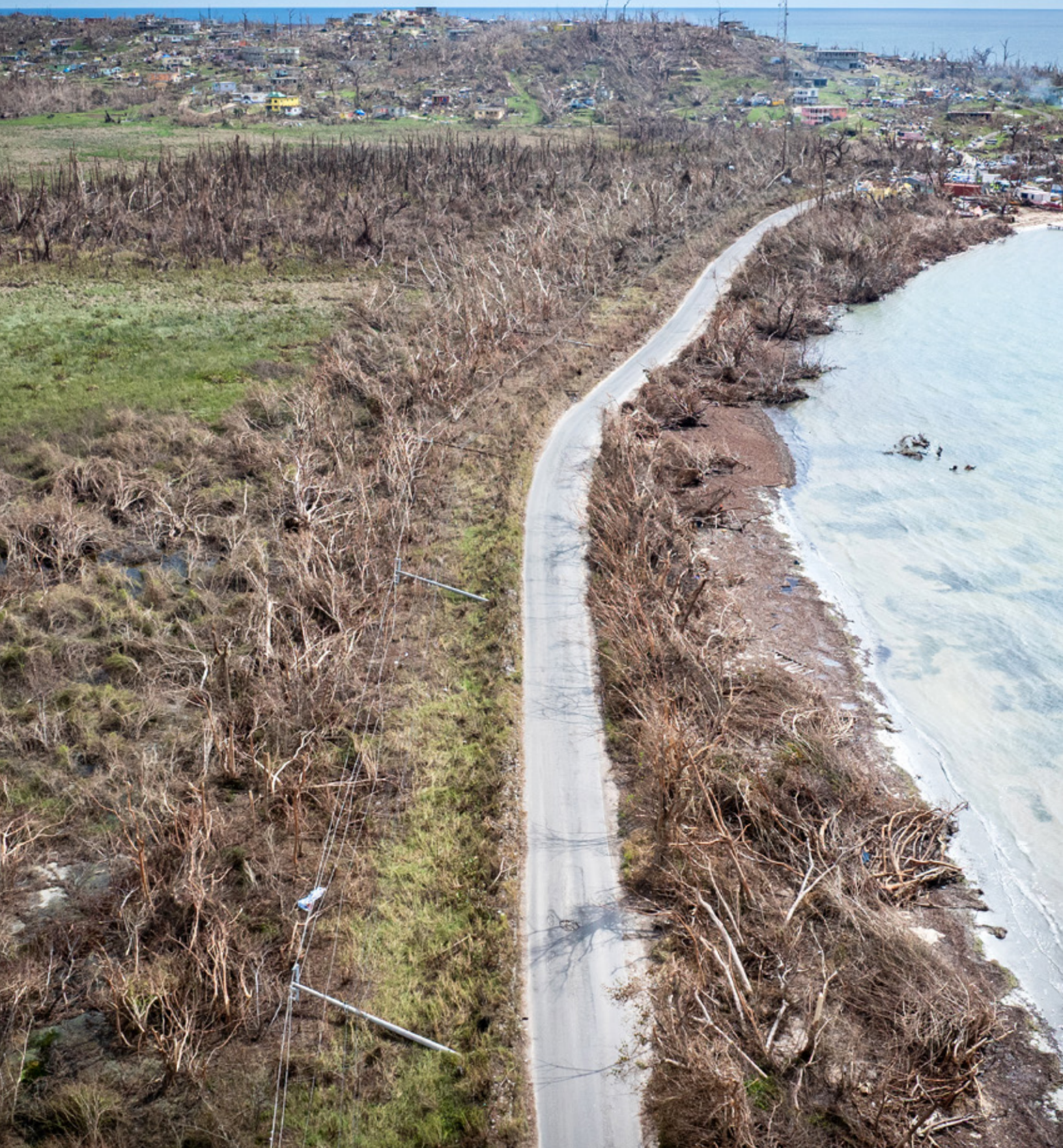
Widespread devastation in Bluefields, Westmoreland caused by Hurricane Melissa
